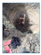
The process started with a single worker digging a huge hole four metres deep (see photo). Then huge piles of sand, stones, metal rods, cement and boulders arrived. The tank was constructed by a team of four within a week.
